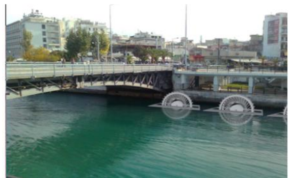
Fig. 7. Horizontal Floating Water Wheels in the Strait of Euripus.
